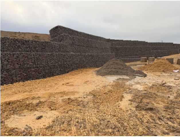
Figures 5 & 6: A Gabion Wall, which allows for animals such as birds to make nests in the gaps in between the rocks.
