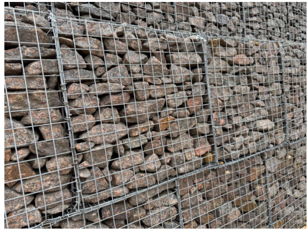
Figures 5 & 6: A Gabion Wall, which allows for animals such as birds to make nests in the gaps in between the rocks.
